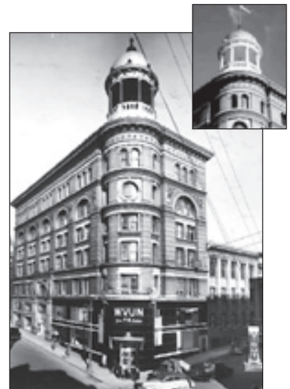
The Dome Building Chattanooga, TN
